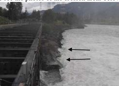
**Type of outage required** – The spillway will need to be on sill (except for Bay 1 which will remain at attraction flow criteria of .5') and fish valves FV4-3 and FV4-4 will be closed to allow the Barge access to the erosion holes. B-Branch is not expected to be dewatered.
